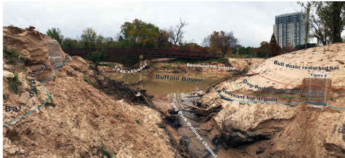
Figure 6. Image looking down Dog Park channel cut
